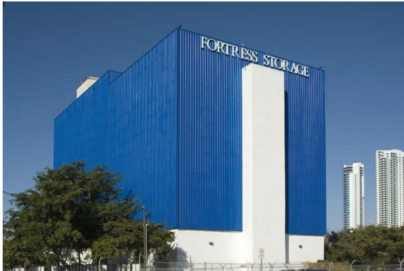
The Fortress building in Miami.
